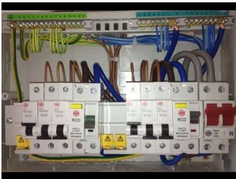
Figure 4.5 Example - internal wiring dressing
